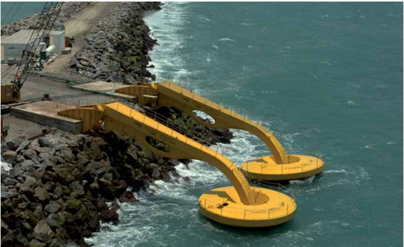
THE FIRST PLANT TO CONVERT WAVE MOTION TO PRODUCE ELECTRICITY IN SOUTH AMERICA WAS TESTED IN THE PORT OF PECÉM, IN THE STATE OF CEARÁ. THE TECHNOLOGY HAS TRACED THE PATH FOR DEVELOPMENT OF OTHER PROJECTS TO HARNESS WAVES TO PRODUCE ELECTRICITY
